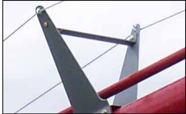
Fig 40 - Cable clamps on truss risers
